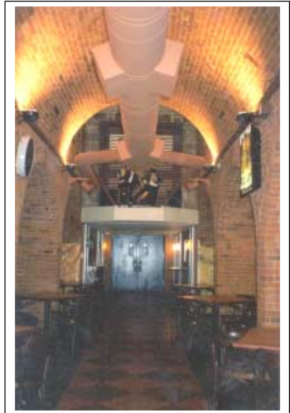
The Cellar – Interior central vault
